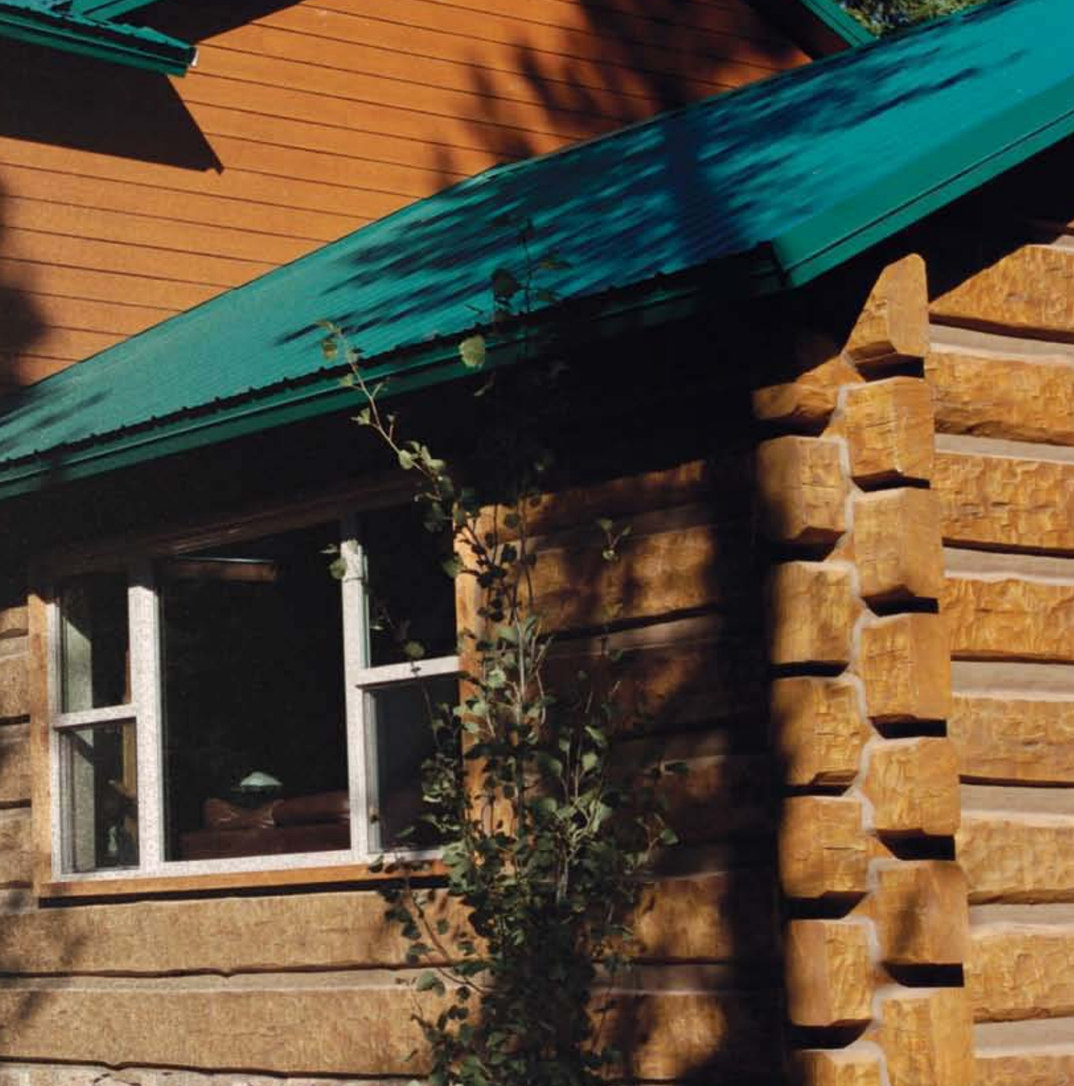
This beautiful log home only looks like wood — it's really concrete. Photos in this article courtesy of Cultured Log Systems.
